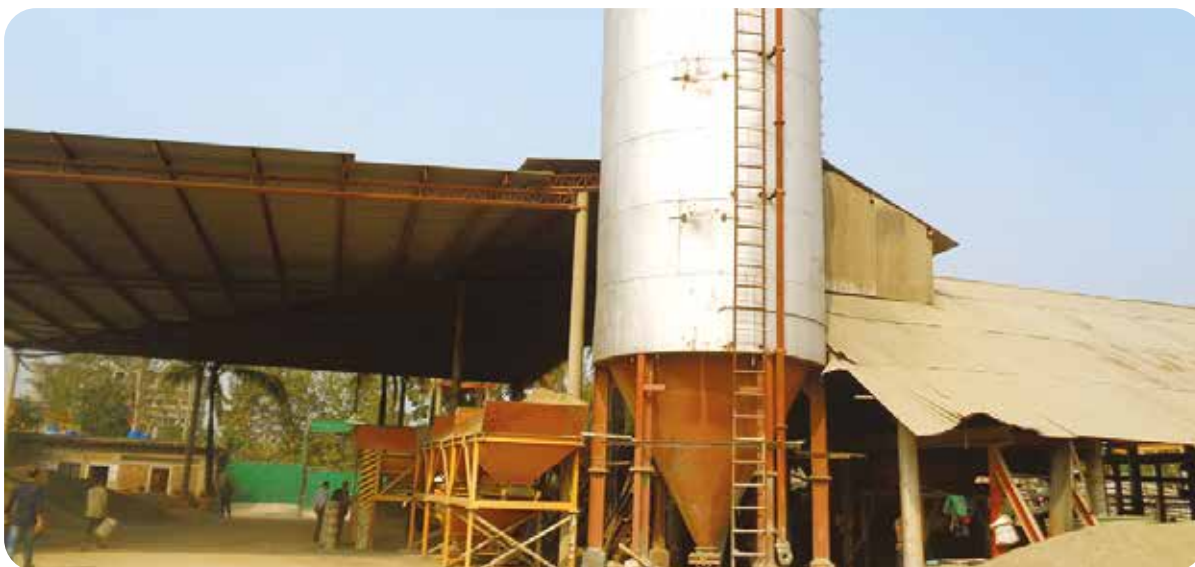
Standard Bank Limited Khulna Branch Financed Glory Poles & Concrete Ltd., Khulna
